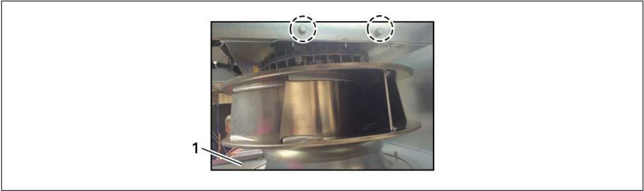
Figure 8.5 Mounting-plate bolt location
