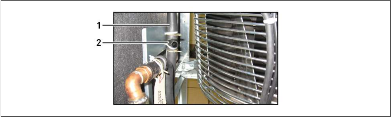
Figure 8.1 Remove the humidifier drain line
